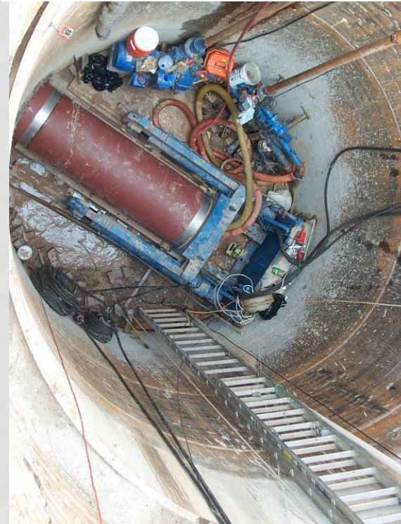
Micro-tunneling horizontally from within the vertical shaft.
