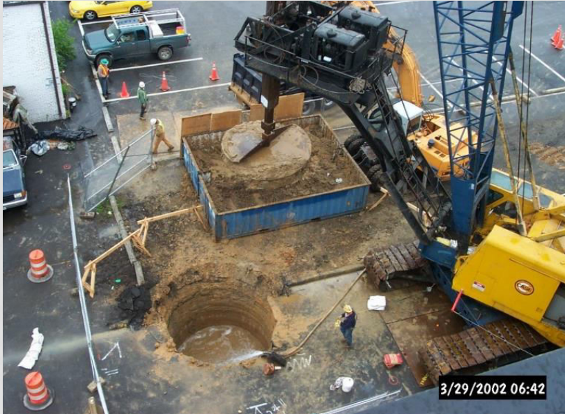
Drilling vertical shafts using an auger.
